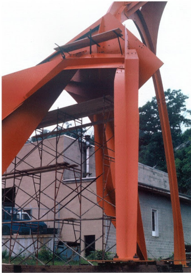
FLAMINGO under construction and in red lead primer at Segre's Iron Works (Photograph by Bob Hicks taken in 1973).
